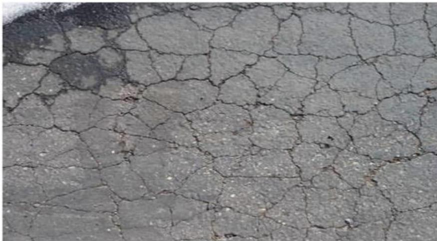
Gambar II.2 Kulit Buaya (Alligator Crack)
