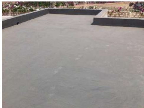
Gambar IV.21 Atap Dak Beton( Google Search, 2021)
