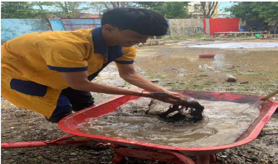
Pencucian Agregat kasar
