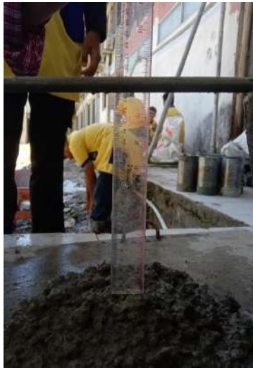
Gambar IV.4 Pengujian Slump Variasi Fly Ash 0%
