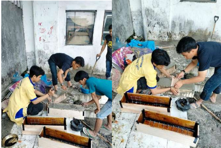
10. Curing (perawatan 28 hari)
