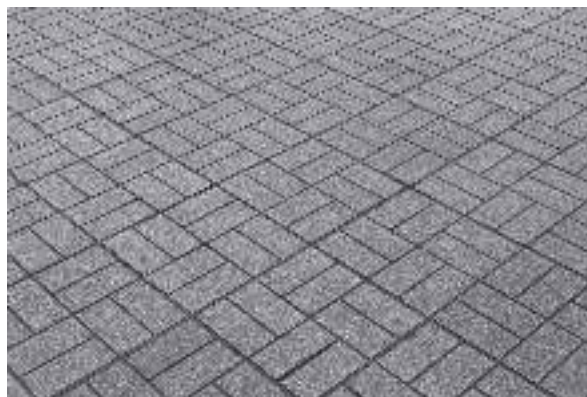
Gambar.IV. 30 concrete Paving (Google,2023)
