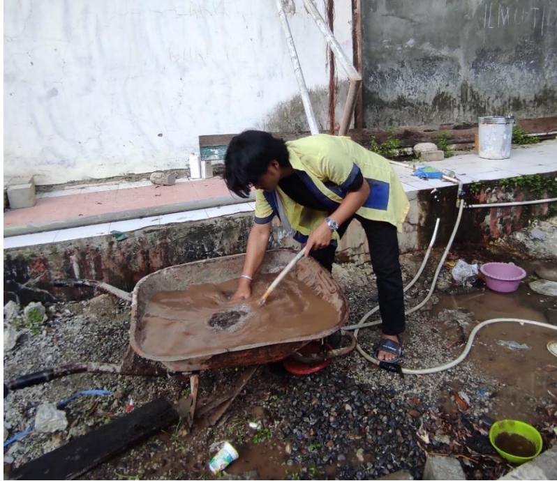
Pencucian Agregat Halus
