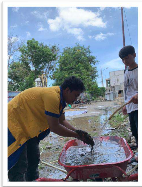
Proses Pencucian Agregat
