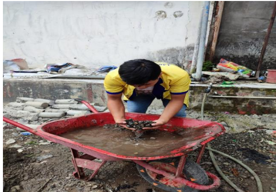
Pencucian Agregat kasar
